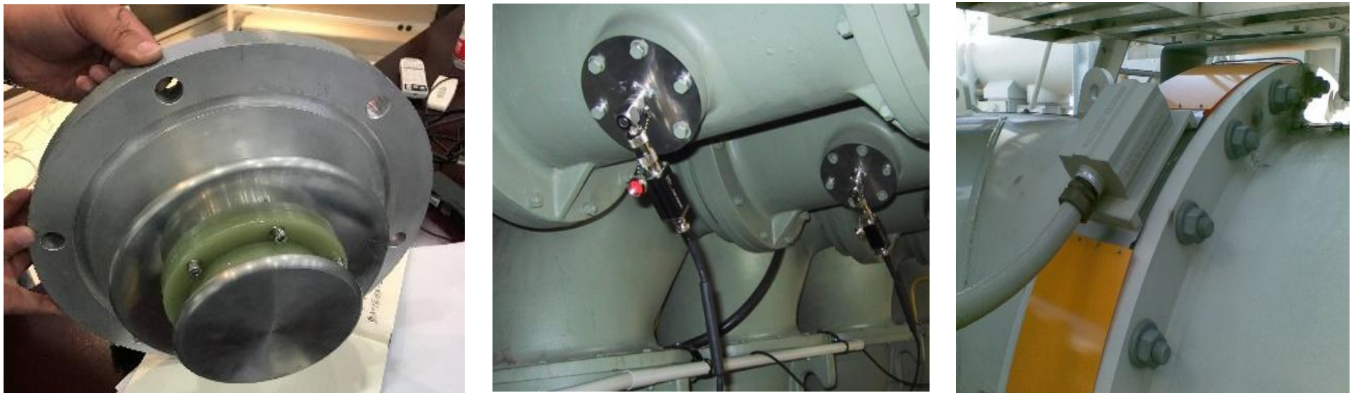
Figure 6 - Examples of GIS/GIL UHF PD sensors
